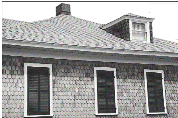
Walker House Baltimore Avenue 1910
