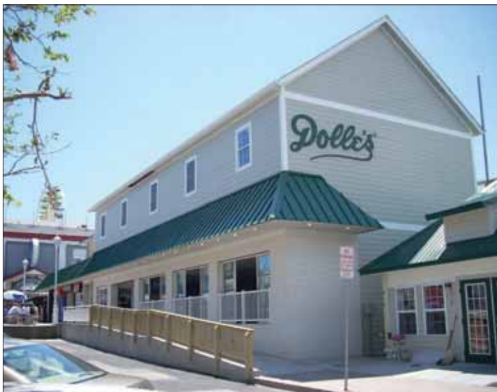
The Cork Bar Building
